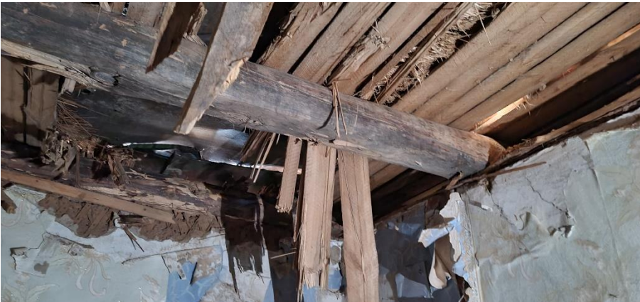
A ceiling was destroyed by rocket impacts. The house is uninhabitable. There are no money and resources to repair it.
