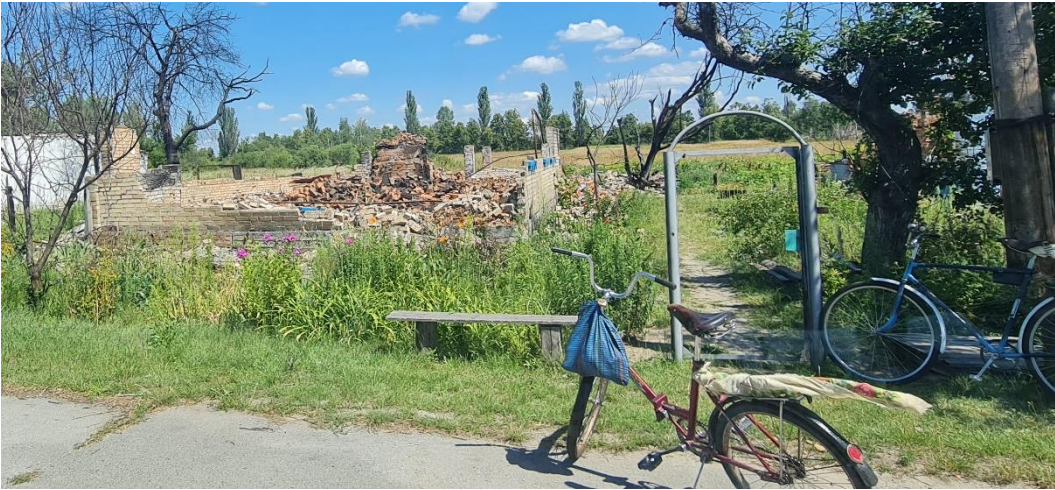
A house totally destroyed.
